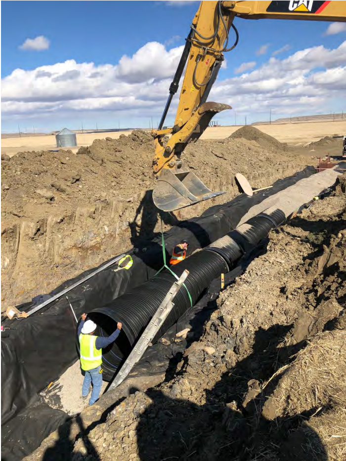
Figure 5-1 Using Pogo Stick in Pipe Haunch Area
