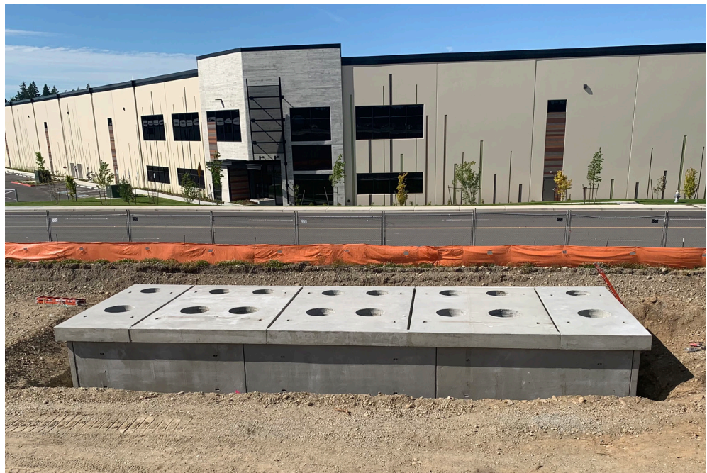
The high-flow StormMix media used in the BioPod meets regulatory requirements to remove TSS, phosphorus, copper and zinc at a fraction of the size of a traditional bioswale.
