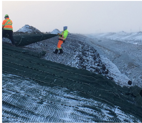
PROPEX Armormax was used to stabilize the side slopes of the channel. Due to delays in construction, project engineers had to overcome challenges such as an accelerated installation schedule and frozen soil.
