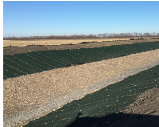
PROPEX Armormax was used to stabilize the side slopes of the channel. Due to delays in construction, project engineers had to overcome challenges such as an accelerated installation schedule and frozen soil.
