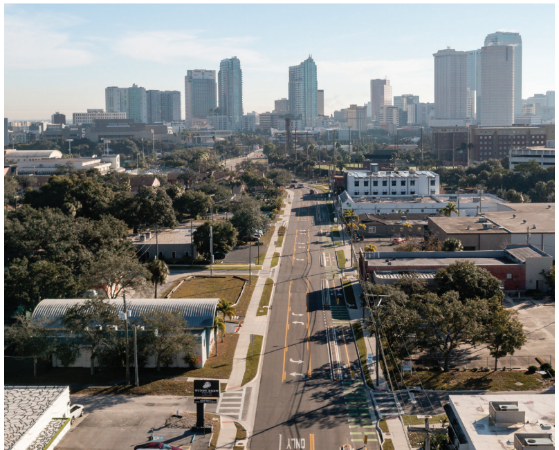
An aerial view of the completed Cypress Street stormwater management project.
