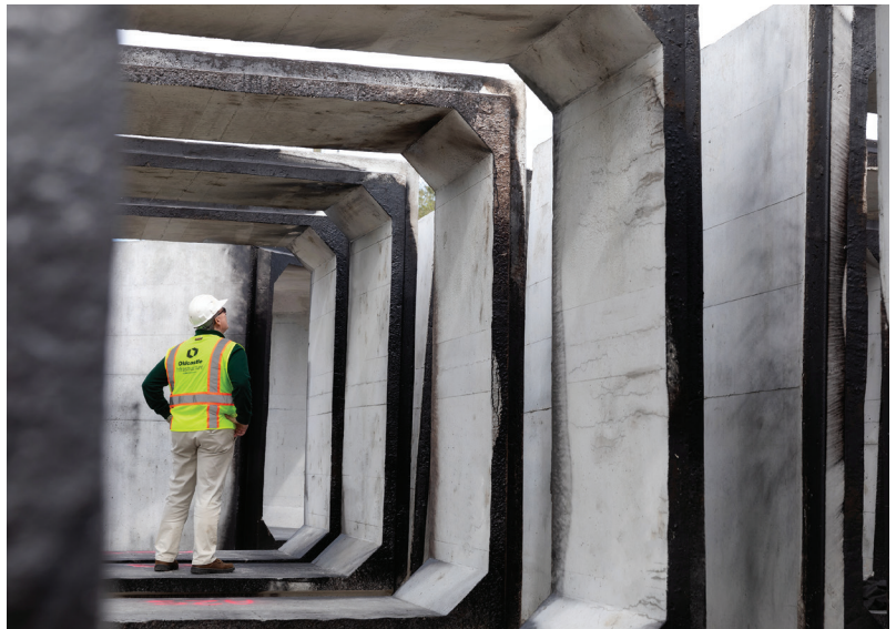
Onsite inspection of box culverts prior to installation.
