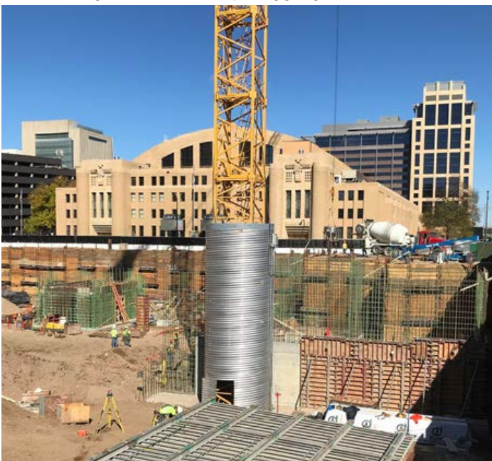
144" diameter HEL-COR® 5 x 1 Corrugated Steel Pipe used as a crane tower enclosure during the construction of a parking garage in an urban area.
