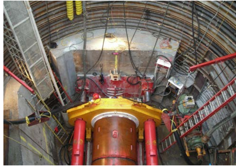
Tunnel Liner Plate Vertical Access Shafts
