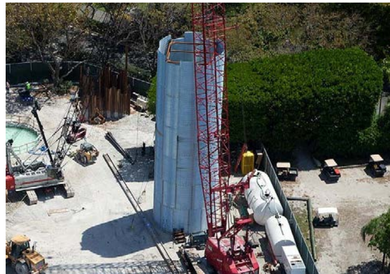
MULTI-PLATE Vertical Shafts are preassembled on site.
