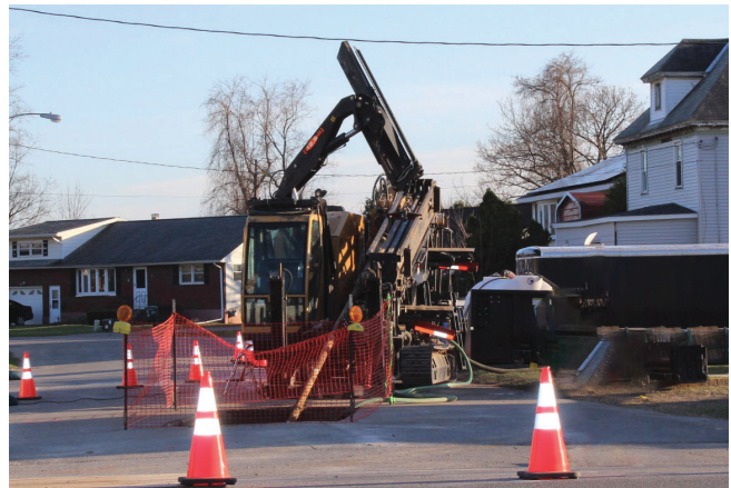
Pressure sewer installation utilizing directional drilling
