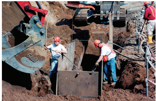
Traditional cut-and-cover method for gravity sewer installation
