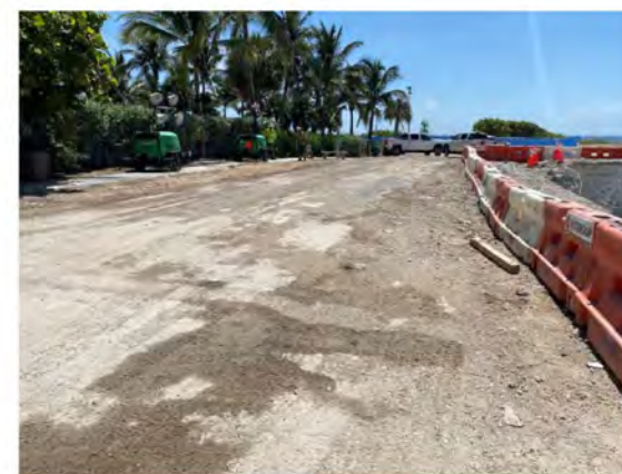
Figure 66- 9K 88 ST Damages Photo 1
