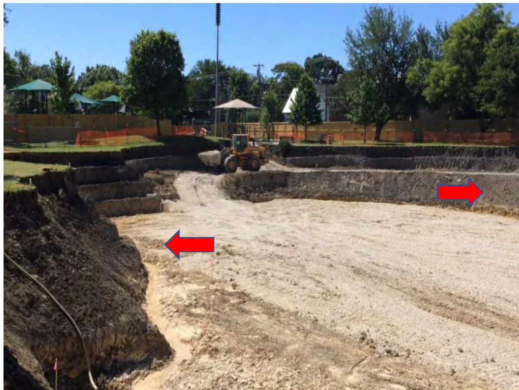
Pumped Water Treated Before Reaching Storm Drain
